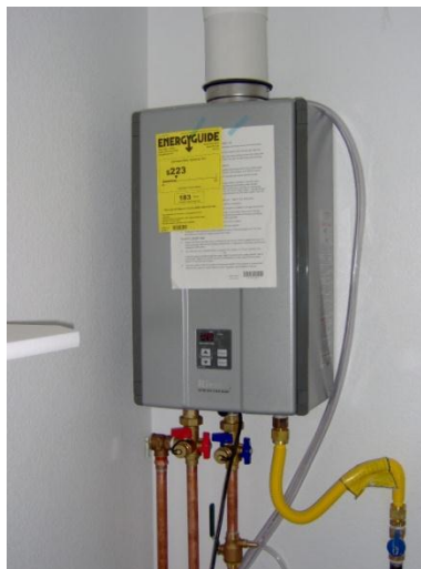
Tank-less Water Heater
