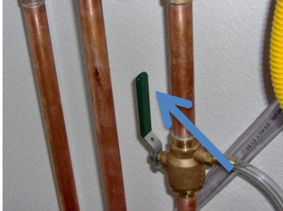
Water valve in “on” position
