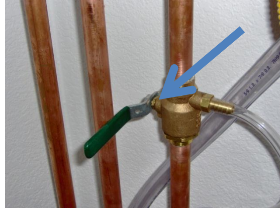
Water valve in “off” position
