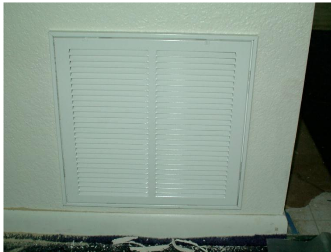
This is the cold-air return. The filter installs behind this cover.
