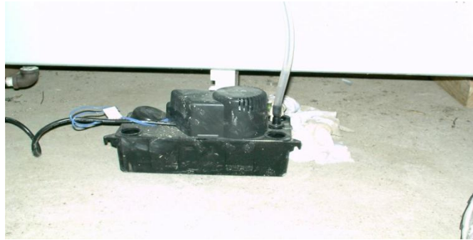
This is the condensate pump located near the furnace.
